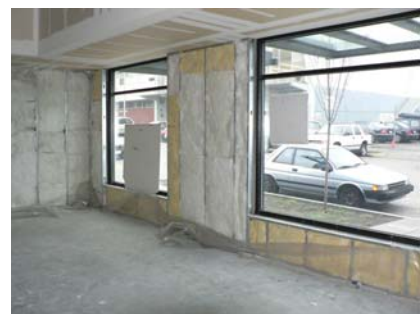
Unfinished interior of new office
