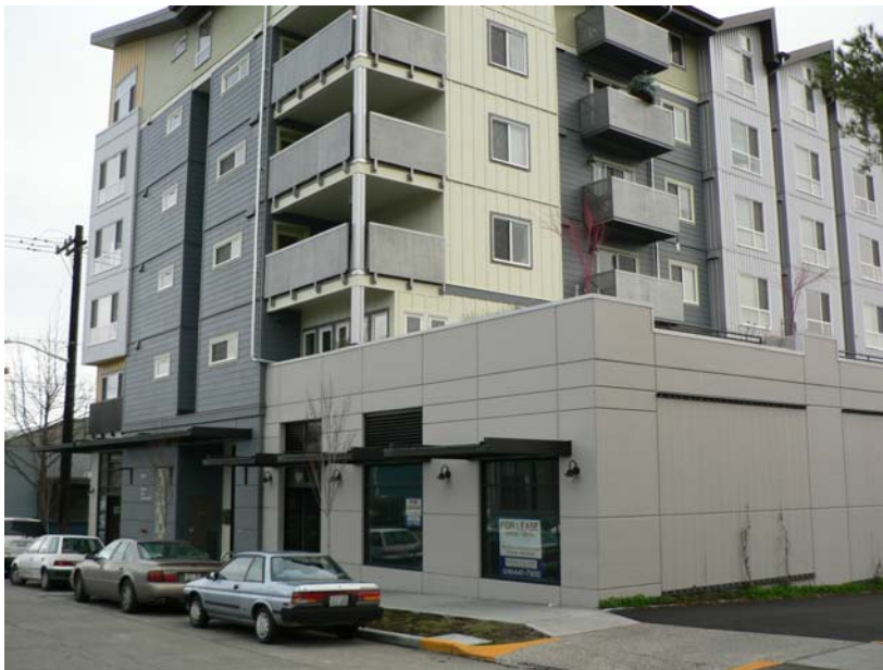
New office is gray portion in foreground of building
